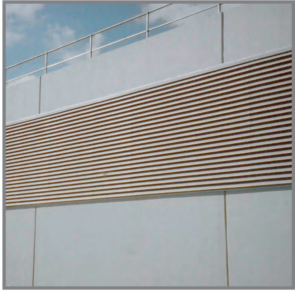
FIXED CONTINUOUS MULLION-LESS LOUVRES ANODISED FINISH
