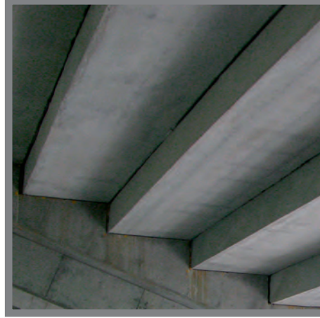
CONCRETE PLATS & SEATING TIER STRUCTURE FAIR FACED CONCRETE
