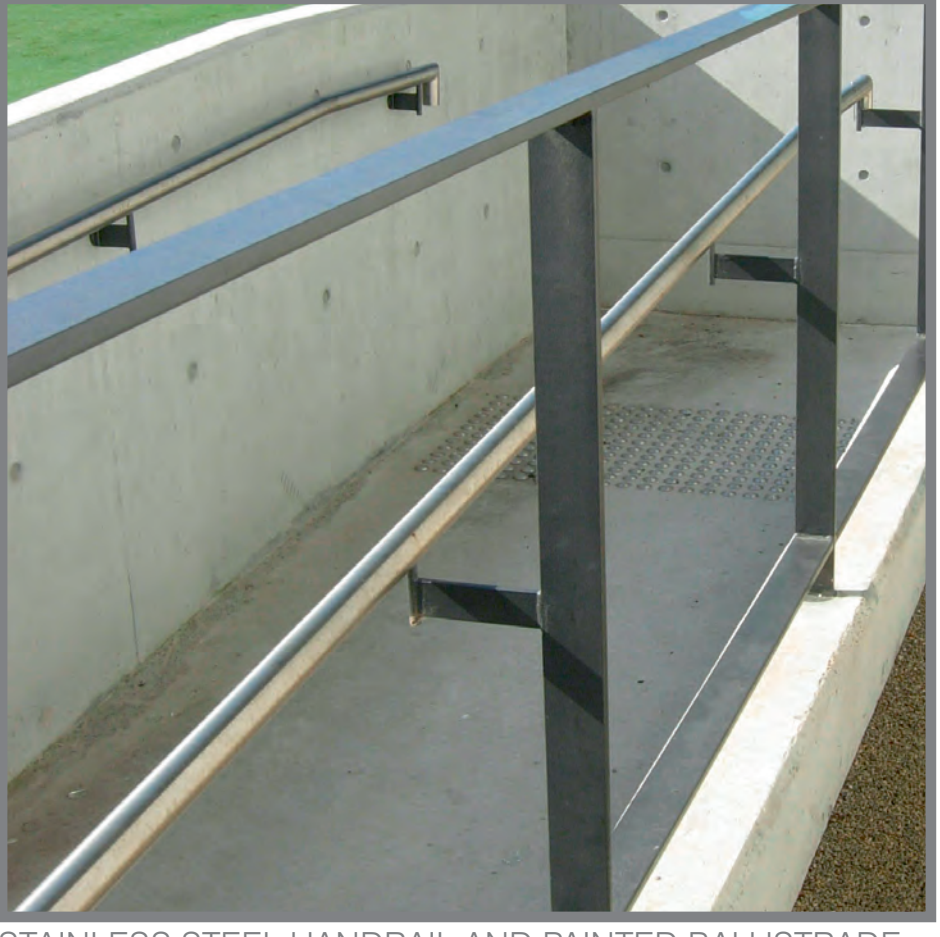
STAINLESS STEEL HANDRAIL AND PAINTED BALUSTRADE
